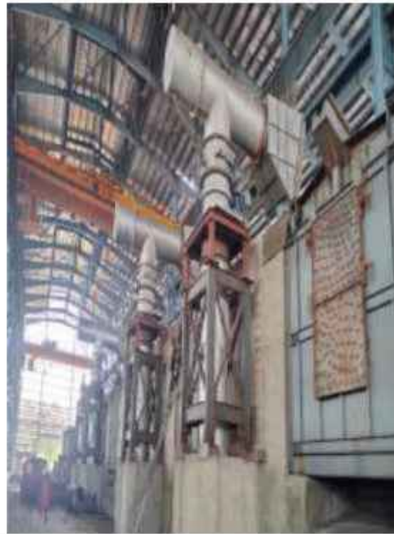
Induction furnace connected with primary hood
