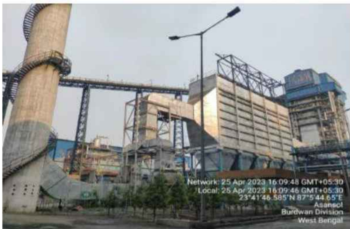
5 field ESP for CFBC Boiler
