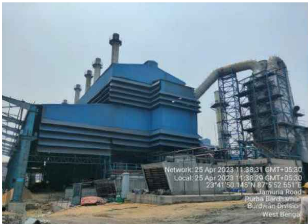
Bag Filter connected with 2x9 MVA SEAF
