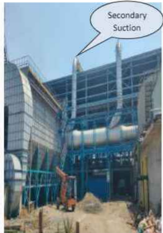
Primary & secondary suction connected with induction
