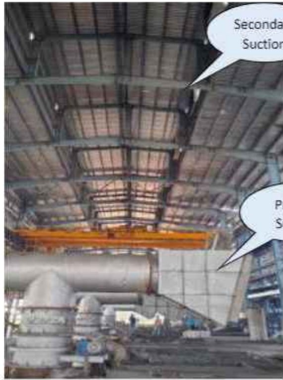
Bag Filter for Steel Smelting Shop
