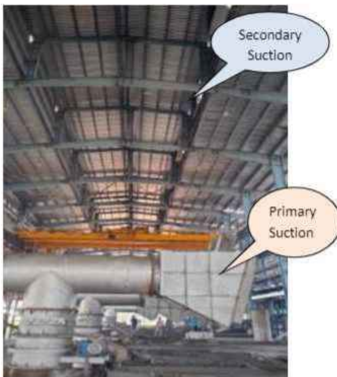
Primary & secondary suction connected with induction
